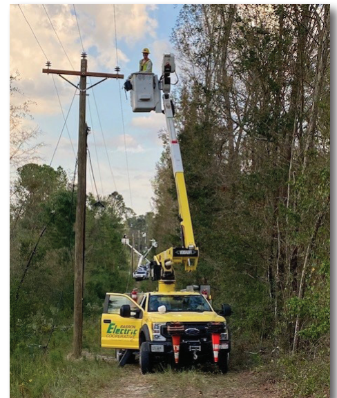
J.T. Gunderson, Barron Electric Lineman, helped rebuild a three-phase line.
