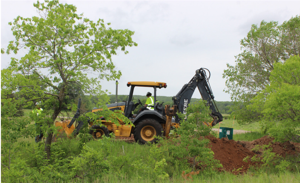
A contractor plows in underground wire.
