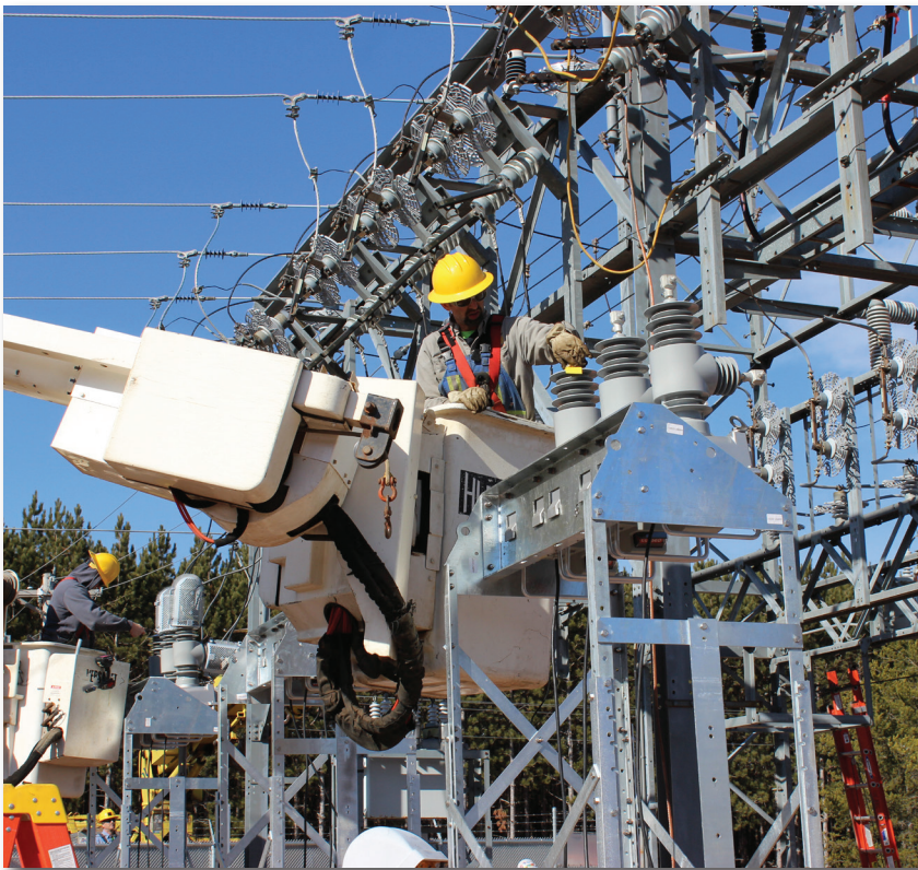
Lineman Ben Brede installed equipment.
