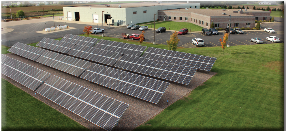
Community Rays was installed in 2014 at Barron Electric's headquarters and provides an affordable option for those members interested in purchasing renewable solar energy.
